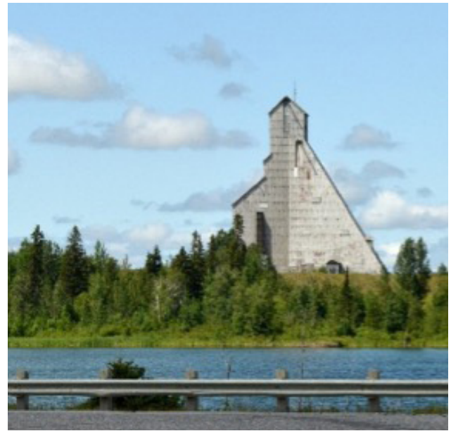
Figure 2: View on the Pearl Lake and shaft of McIntyre Mine (Timmins). Photo: K. Bulcewicz
