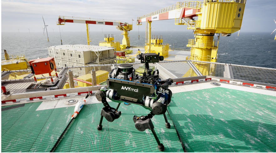
Fig. 1: The quadrupedal robot ANYmal was deployed for autonomous inspection and surveillance on a wind energy HVDC converter platform in the North Sea.
