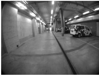
(c) NAV: parking garage
