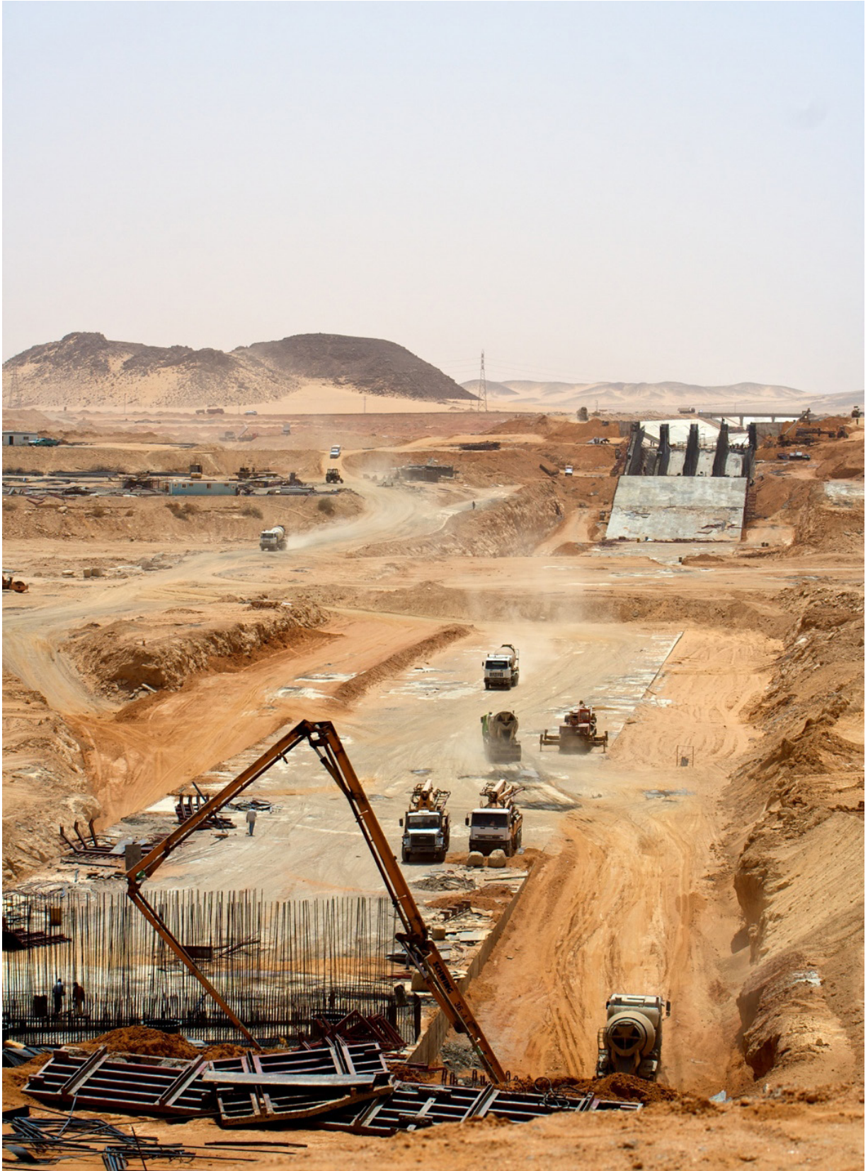
Construction of the Toshka Spillway, the first infrastructure of the project, originally dug as a siphon for Lake Nasser, 1984 (Wikipedia Commons).
