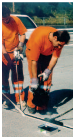
Fig. 1: Joint installation on the trial road section.
