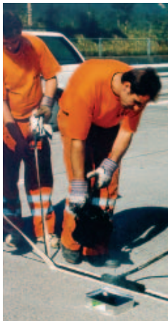
Fig. 1: Joint installation on the trial road section.
