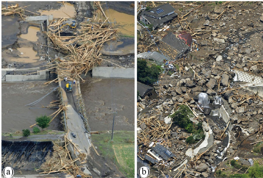
Figure 2.11 2012 flood in Taketa (prefecture Oita in northern Kyushu, Japan), (a) LW accumulation at a bridge (Photo: dailymail.co.uk ) and (b) debris flow with LW (Photo: democraticunderground.com )
