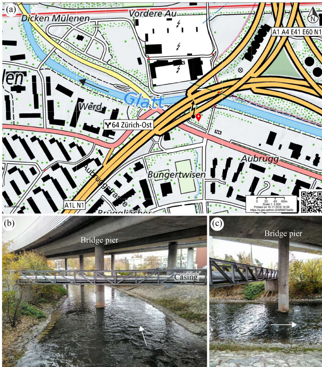
Figure 6.1 (a) Map of River Glatt in Zurich (swisstopo 2017), (b) and (c) circular bridge pier
