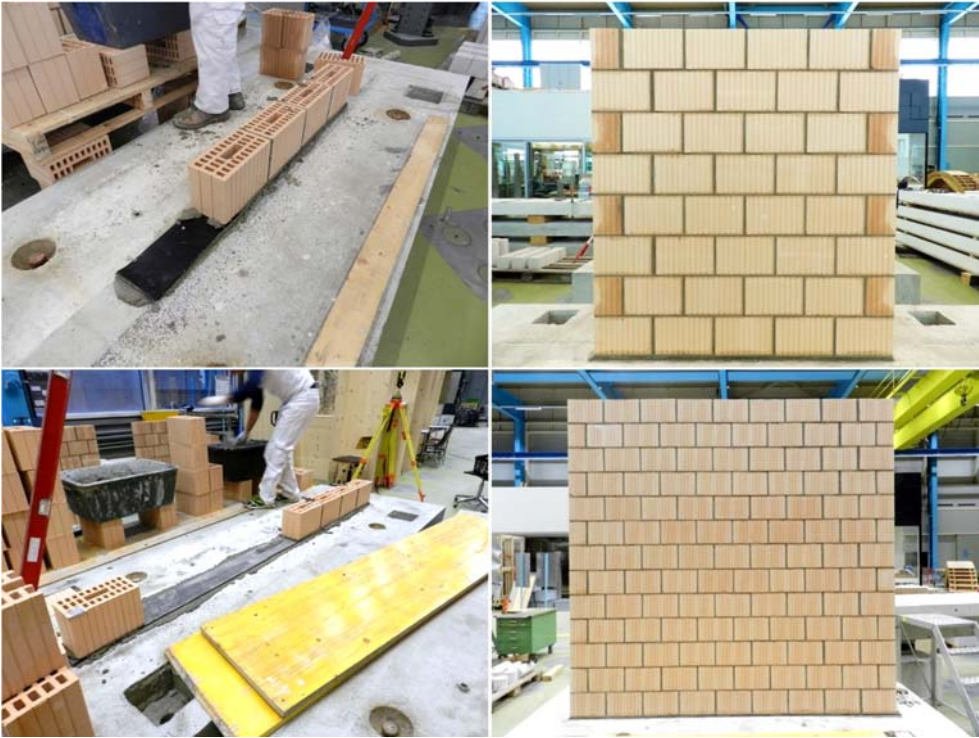
Figure 3-27. Construction of the specimens
