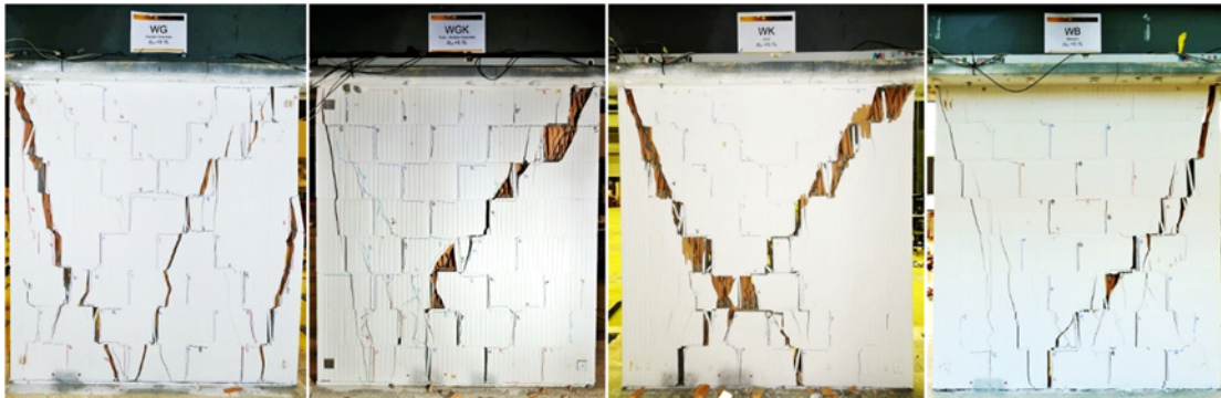
Figure 3-36. Final crack patterns of the specimens in the preliminary testing phase [40]
