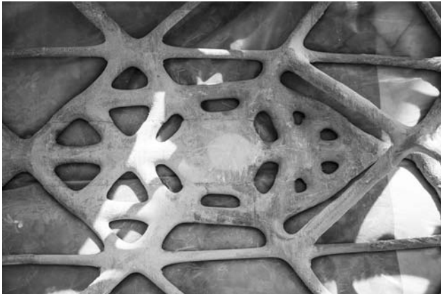
Figure 4: The complex concrete “skeleton” displaying an intricate network of narrow tubes. (DBT, ETH Zürich, 2017)
