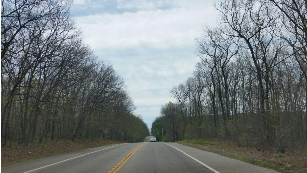
(a) Two-lane rural highway in Connecticut. (US44)
