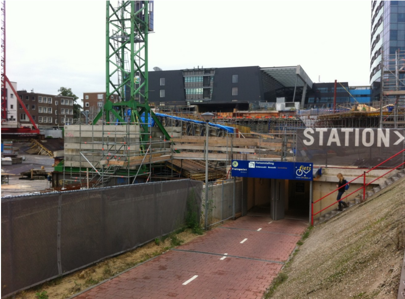
Figure 14.6: Construction at train station Arnhem, Gelderland, Netherlands. Photo by D. Levinson.
