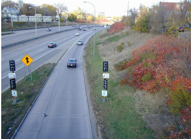
Figure 6.10: Ramp meter, 4th Street at I-35W Northbound, Minneapolis. Photo by D. Levinson.
