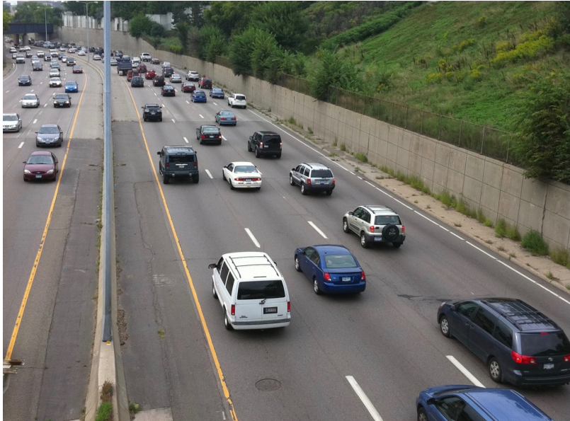
Figure 6.2: I-94 in Minneapolis. Photo by D. Levinson.
