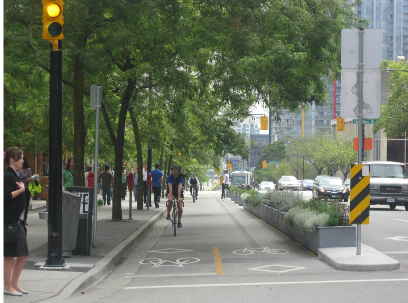
Figure 3.8: Protected bike lane in Vancouver, British Columbia, Canada. Photo by Wes Marshall.
