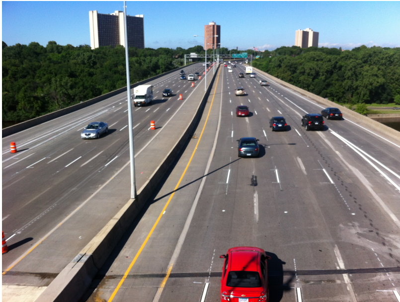
Figure 6.11: I-94 Mississippi River Bridge. Photo by D. Levinson.
