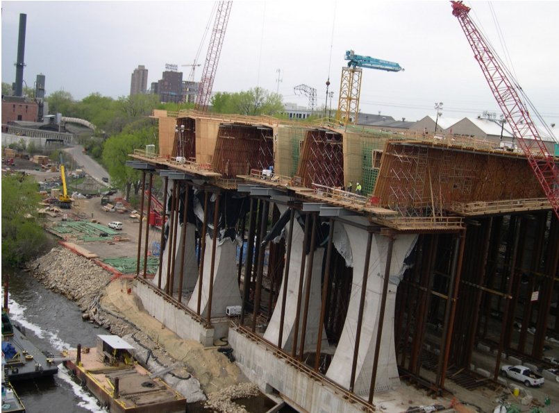
Figure 9.4: I-35W Mississippi River Bridge under construction. Photo by D. Levinson.
