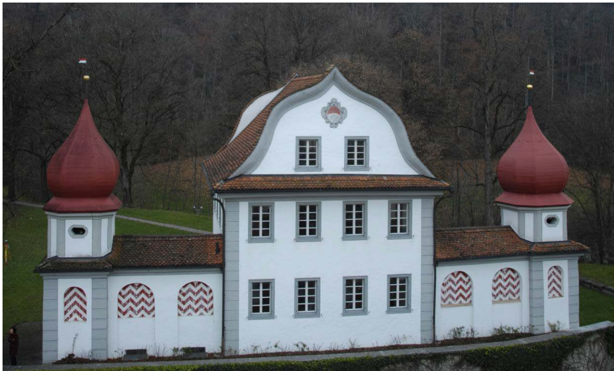
Figure 6-23: Front view of castle Landenberg. The image was acquired with our UAV-system.
