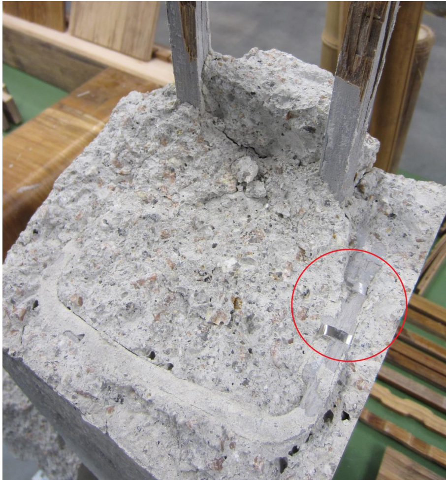
Fig. 165 Intact steel cable ties after shear failure of the concrete beam sample from B3b2 series
