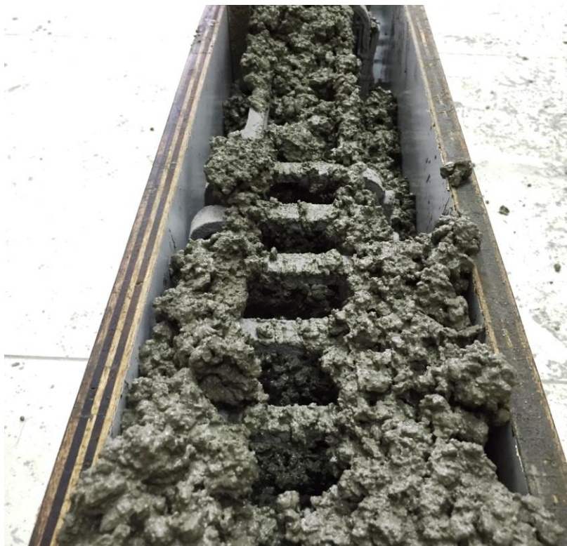
Fig. 154 Pouring concrete mix in three stages into the wooden mold
