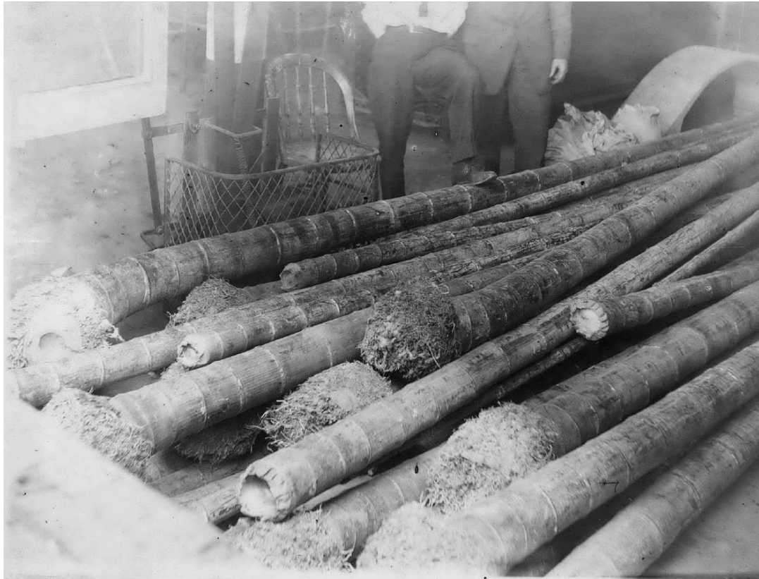
Fig. 23 Bamboo poles used by Hou-kun Chow at MIT in 1914 for reinforcing concrete beams (Chow 1914)
