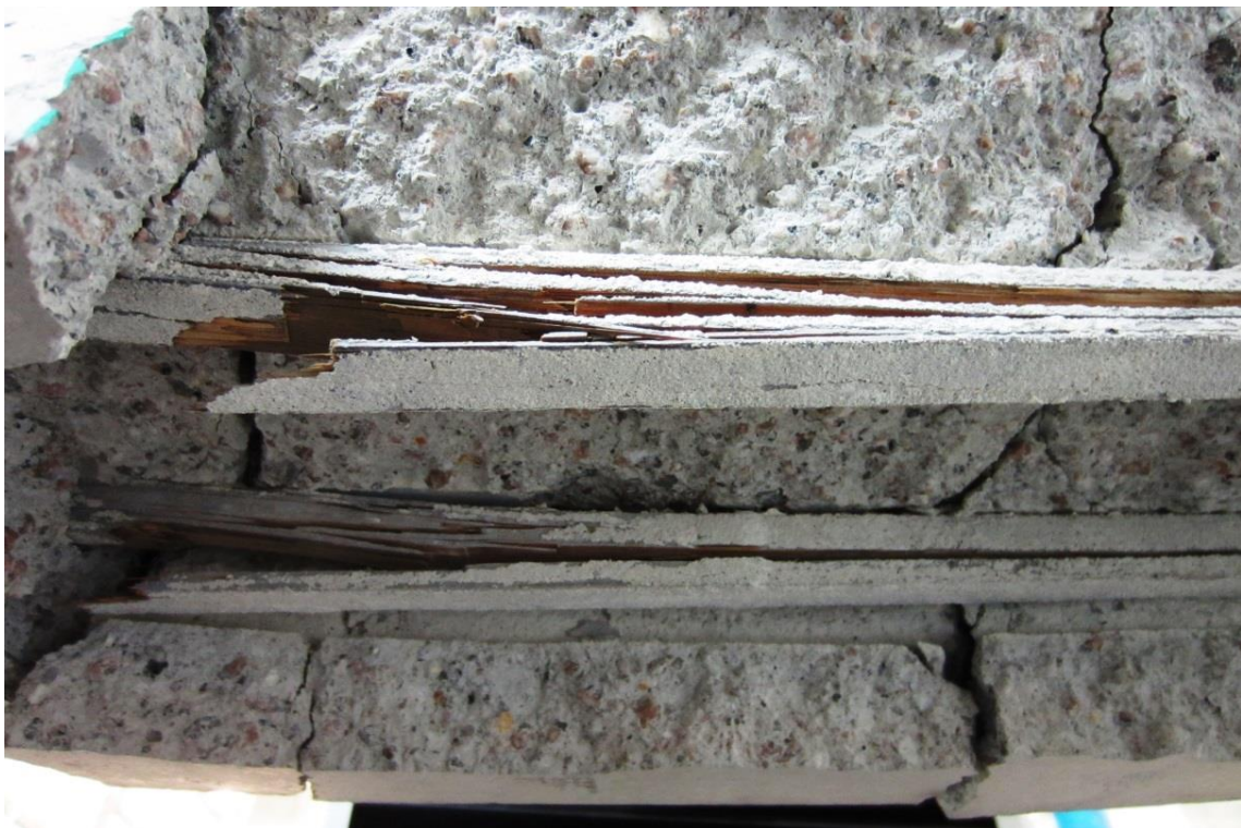
Fig. 167 Tensile failure of the BVC reinforcement at the tension face of the concrete beam sample
