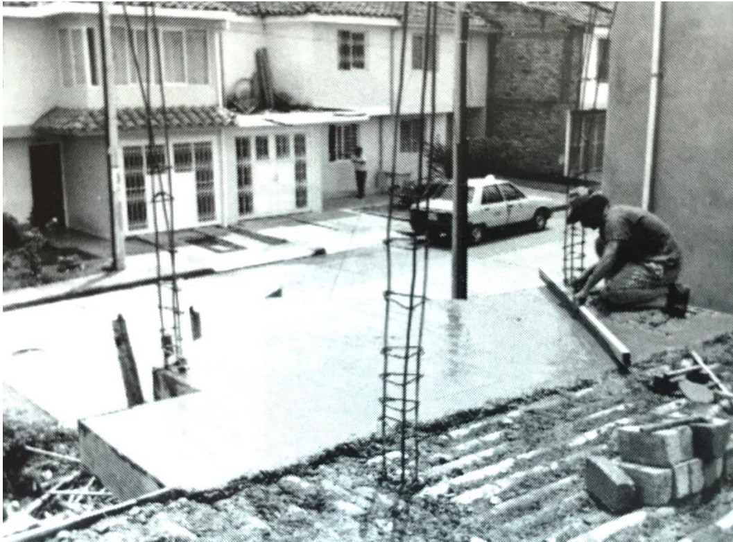
Fig. 37 Bamboo reinforcement for concrete floors of housing projects in Colombia (Hidalgo-Lopez 2003)
