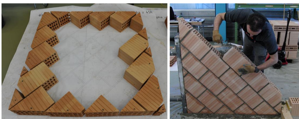
Figure 3-16. Construction of the wallettes with inclined bed joints
