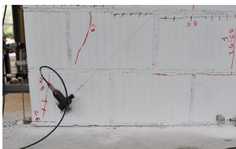
Figure 4-11. Separation of Wall T7 from the foundation due to the rocking motion of the wall
