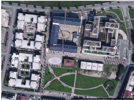
Fig. 1: Aerial view of the social housing in Cremona, Italy.
