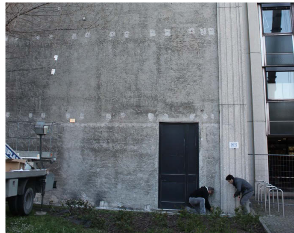
Fig. 10: individuation of the bubble and entire anchoring system set-up on the test façade.
