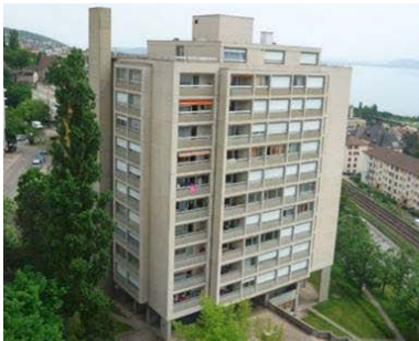
Fig. 3: Building image (current status).
