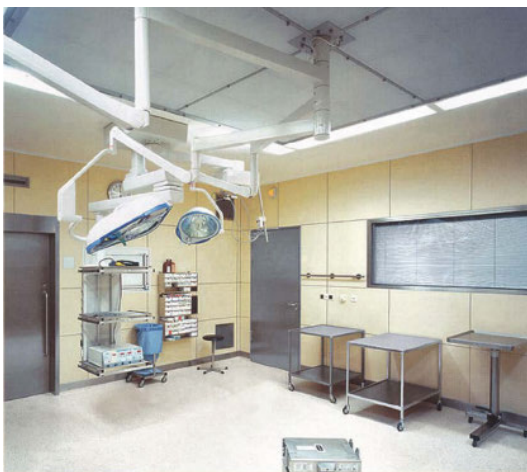
Fig. 11: Operating theatre, Berlin, Germany (Product: "Hydrotec" tiles, photocatalytic surface with antibacterial effect) [4].
