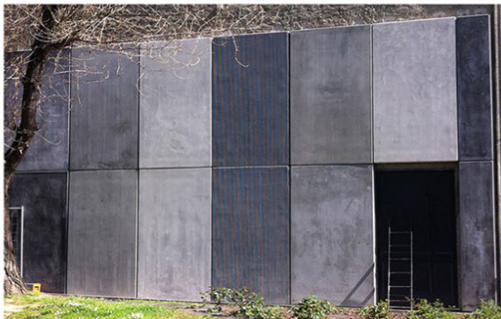
Fig. 12: Installation and levelling of the panels on the test façade.
