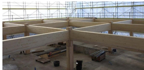
Fig. 1: Post-tensioned timber frame.
