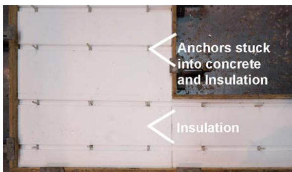
Fig. 7: Thermal insulation as a moulding / EBB.
