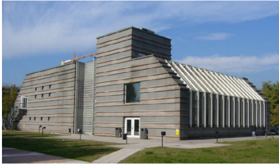
Fig. 2: Brescia Smart Campus Building, Italy.
