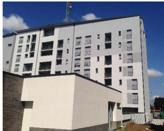
Fig. 3: View of the south façade of the building.
