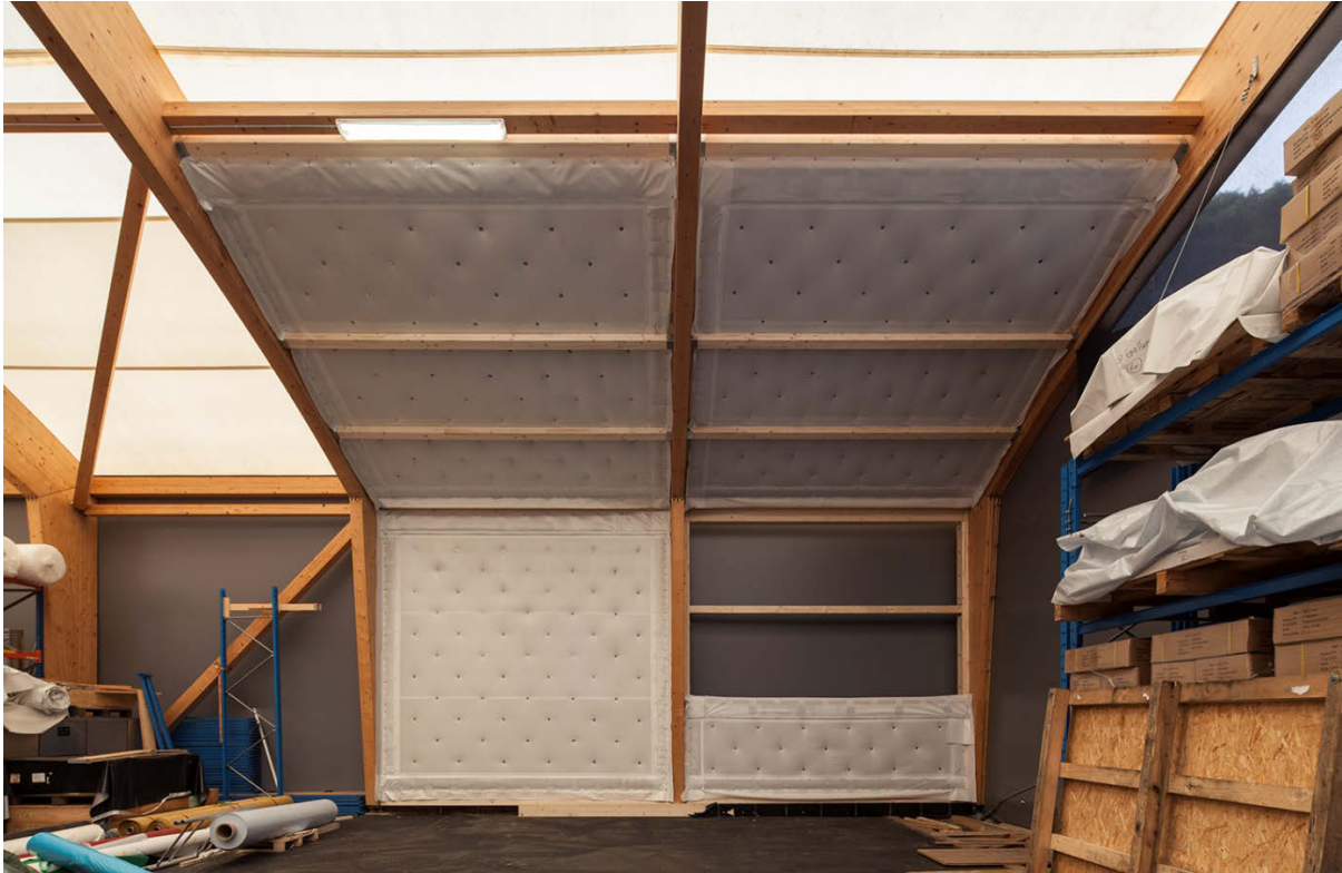
Fig. 2: Prototype of the textile retrofit system.
