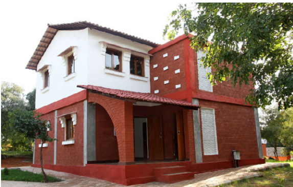
Fig. 5: Demonstration house made with ternary blend cement LC 3 in Madhya Pradesh, India.
