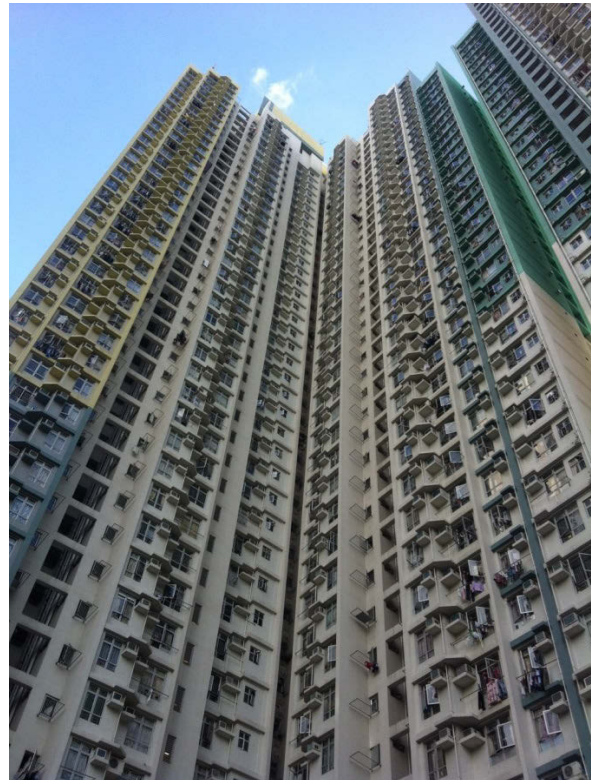
Fig. 3: Residential high riser Hong Kong, photo © Ferdinand Oswald 2013.
