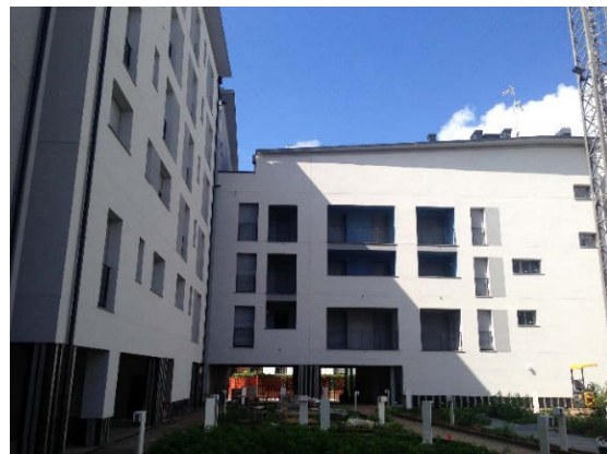
Fig. 4: View of the east and north facades of the buildings in the courtyard.
