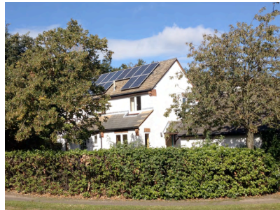
Figure 3: PV panels (2.7 kWh peak) on Participant's roof facing south-east, shaded by trees, at 42 degree pitch
