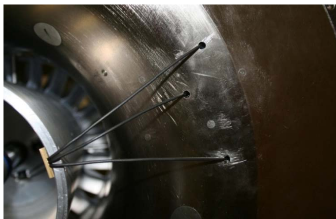
Fig. 5.47 The Three Accelerometer Cables are fed through the Impeller Shroud and connected to the M12 Module.
