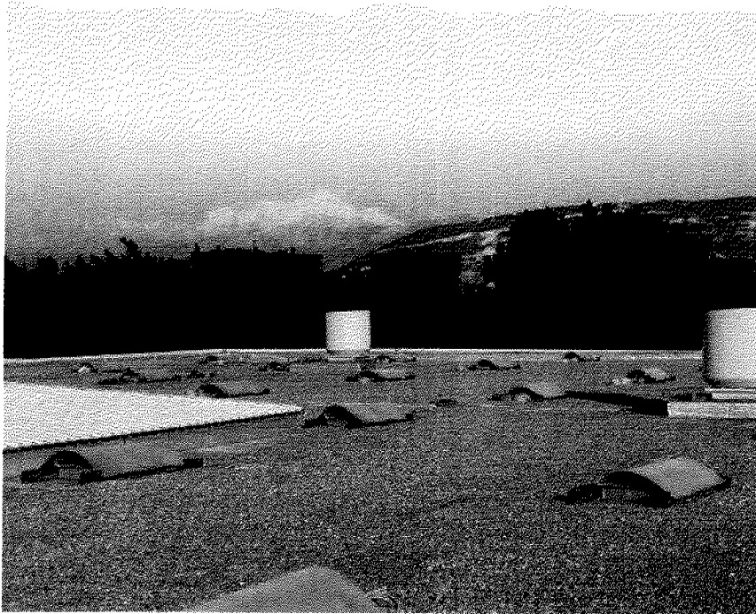
Figure 3.9: Air shower array mounted on the roof of the surface building
