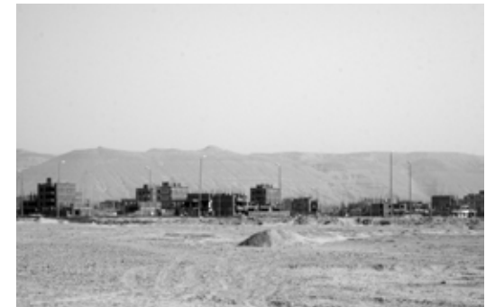
New Assiut under construction, Egypt
