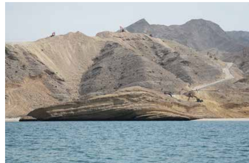
Construction for a coastal resort
