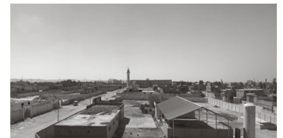
Beni Ghaleb industrial park outside of Assiut, Egypt
