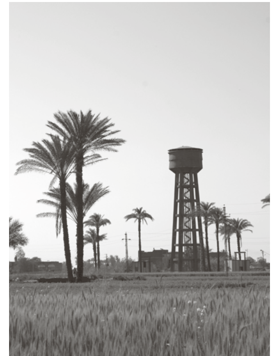
Water tower in Assiut Governorate, Egypt
