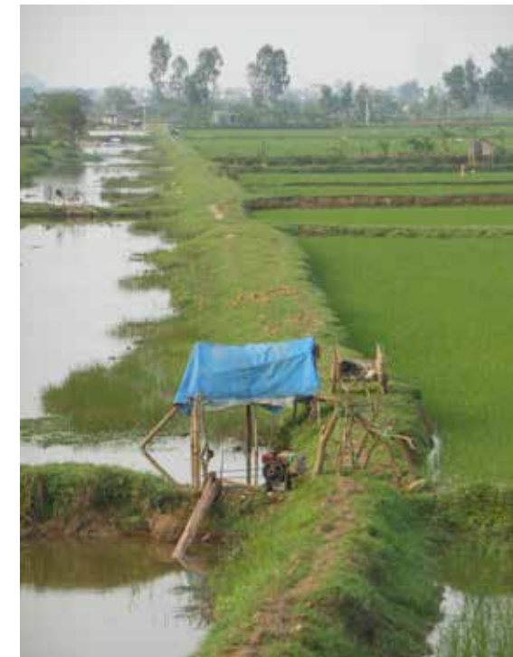
Drainage canals of the polder Bac Nam Ha
