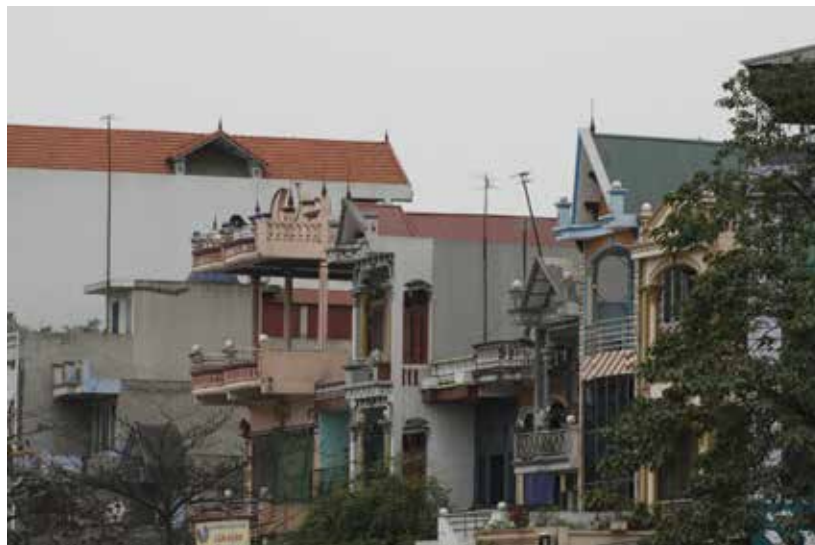
Individual facade treatments along the street front
