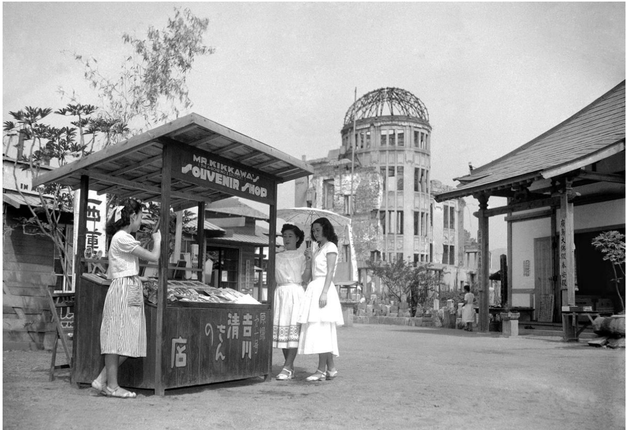
Fig.130: Six years after an atomic bomb was detonated above this spot in Hiroshima, a souvenir shop stands in the street near the shattered dome of the Industry Hall. The shop is operated by Kiyoshi Kikkawa, who was injured in the blast, 3.8.1951, (photo retrieved through: < http://www.theatlantic.com/photo/2014/03/japan-in-the-1950s/100697/ >, last access 9.11.2014)
