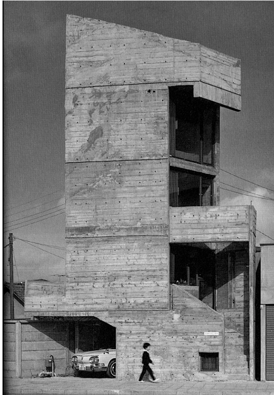
Fig.288a): Takamitsu Azuma, Tower House , 1966–1967, Tokyo, outside view, photo, (in: Saitama 2014)
