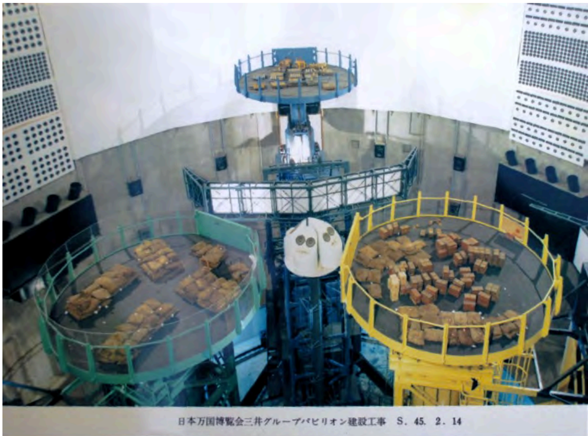
Fig.277: Katsuhiro Yamaguchi et al., Space Theater , Mitsui Group Pavilion, Osaka Expo '70, 1970, weight test on three rotating platforms in the dome shaped main room, center, to the left and right: speaker system, photo, (in: Mitsui Pavilion Papers, Mitsui Bunko (Archives), Tokyo)
