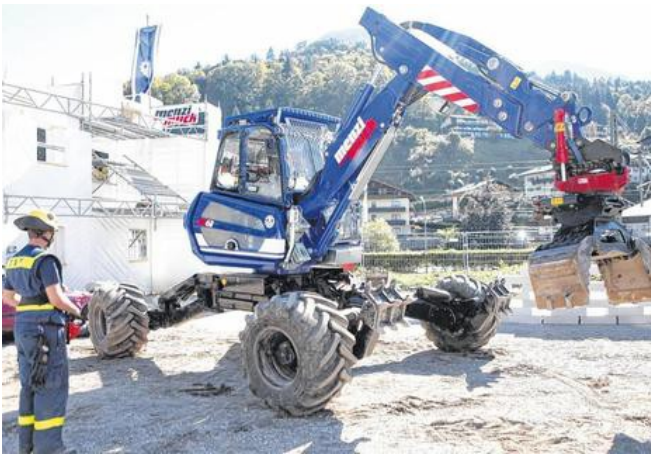
Fig. 2. Typical setup for teleoperation of construction machinery for disaster recovery work (picture THW)
