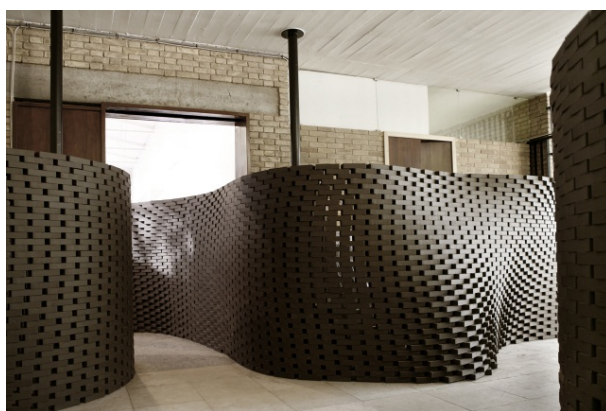
Figure 65. Structural Oscillation : (top) Overview of the 26 individual wall segments; (bottom) image of final installation, the individual wall segments are combined to create a continuous wall.
