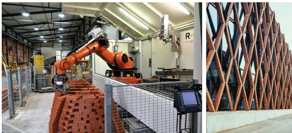
Figure 70. Gramazio & Kohler Architects, Façade Ofenhalle, Pfungen, 2012: (left) robotic assembly process of façade members; (right) installed façade.
