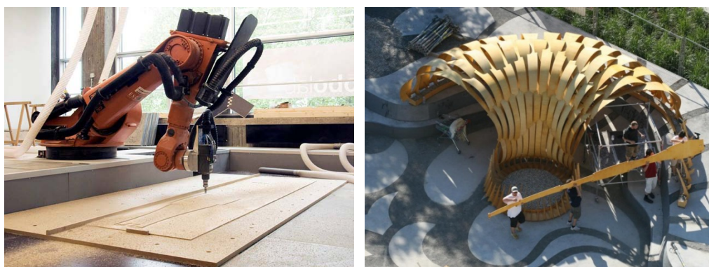
Figure 4. ICD/ITKE Research Pavilion: (left) robotic milling of plywood plates; (right) assembly of planar plywood plates to a bending-active system.
