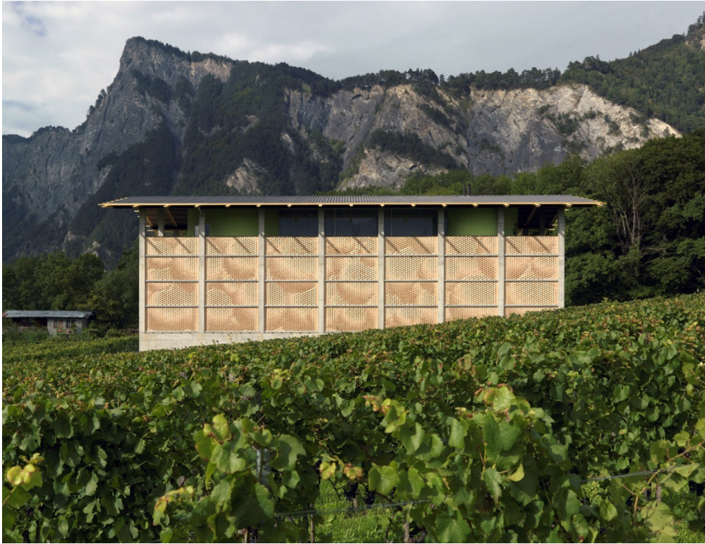
Figure 43. Experiment 2: View of installed façade of the Gantenbein winery (see Section 4.5.6).
